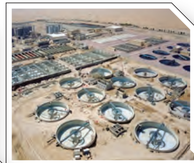
Sewage Treatment Plant
