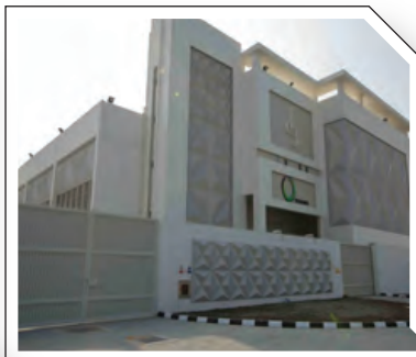
Substation Near Ibn Battuta Mall
