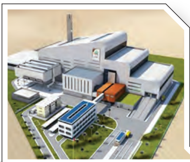
Khazna Data Center
